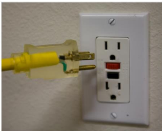
Level 1 Charging - Standard House Outlet
